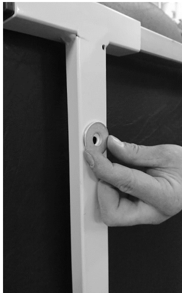
Figure 3: Shims as support for wall mounting
